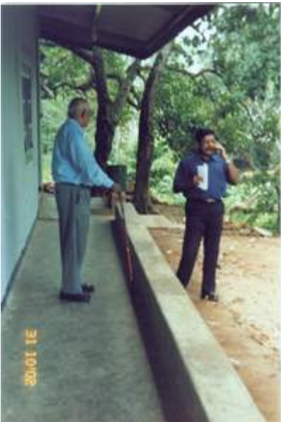
Laboratory Roof - urgent repairs required
