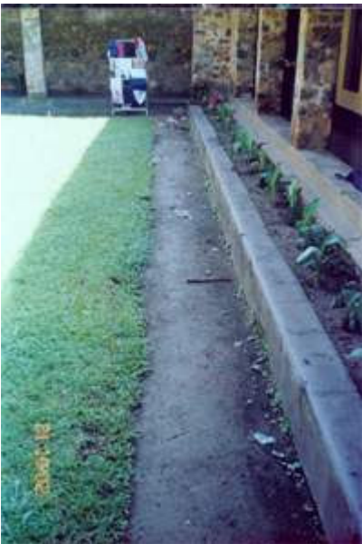
Mahen goes round with maintenance Supervisor
